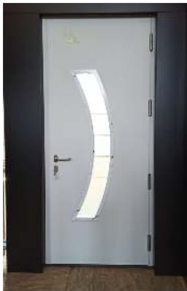
C2 Internal view
